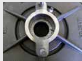
New rope packing installed
